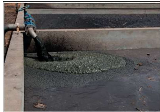
Loading of an unplanted sludge drying bed
