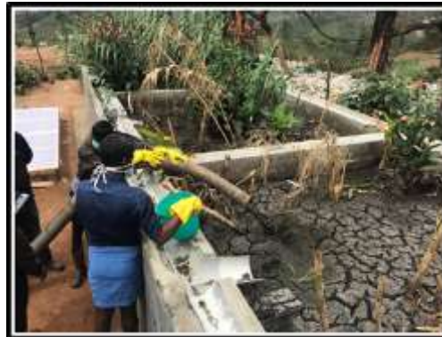
Discharging Fecal Sludge in planted sludge drying bed
